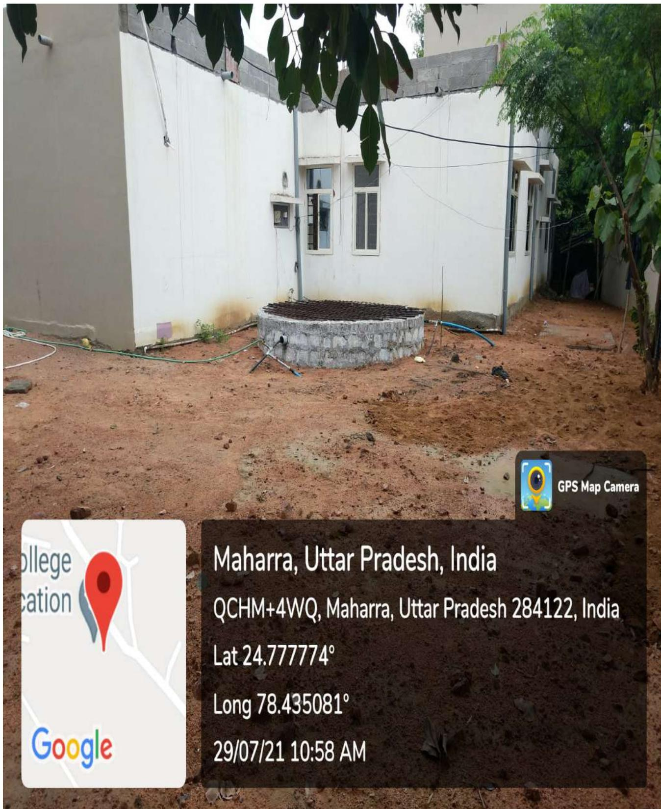
Water is collected through pipes which are connected to the roofs of the entire campus. The collected water is drained through drain system created in the peripheral of the campus. The water is finally collected to rain water harvesting.
